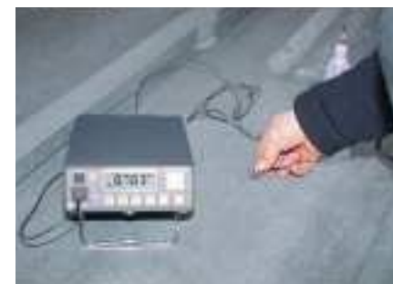
Fig.2: Thickness measurement with the ultrasound thickness measuring unit.
