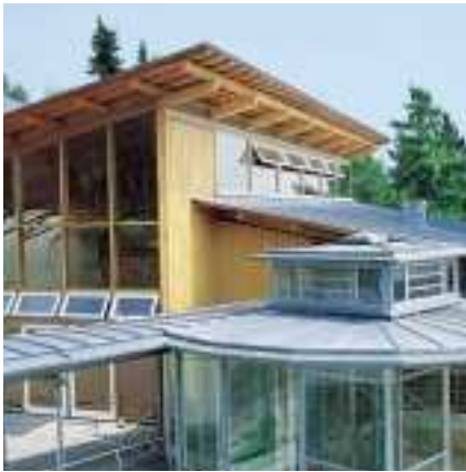
Fig. 5: Example of a “grey water” utilization system: “House in the Vineyard” community centre in Markdorf, Germany.
